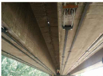
土木工程加固 Civil engineering reinforcement
